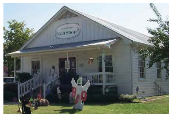
Clapboard siding and metal roofs over porches are appropriate materials for Old Coppel.
