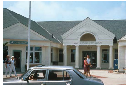
Vertically oriented projecting bays are used here to break up the main horizontal roof plane and articulate the primary entrance of the building.
