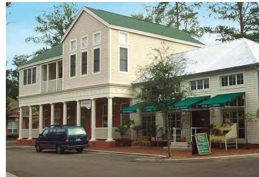
This building utilizes a varied pattern of building segments, porch columns and awnings to break up the massing into a human scale.
