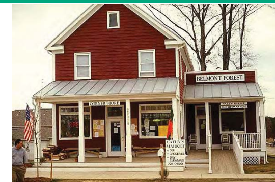
This building is consistent with 2.5 story maximum height for Old Coppel. The porch canopy and the adjacent one-story wing further reduce the perceived height.
