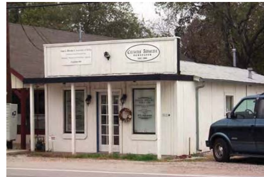
As indicated by the historic photographs on Sheet 2, there is a historic precedent for parapet wall screening gable roofs in Old Coppel, although few examples have survived.
