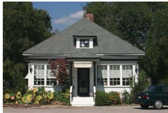
Pyramidal roofs are an acceptable roof form and are common for bungalows.
