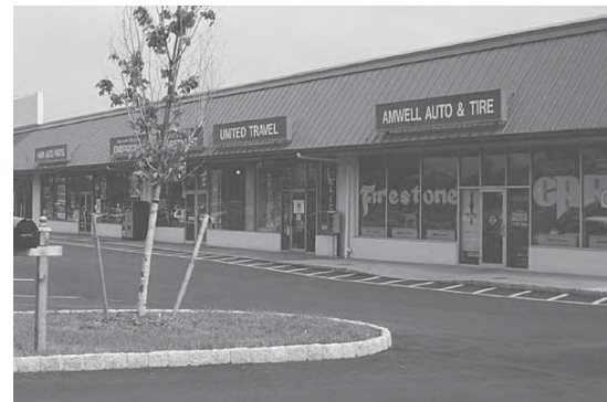
The flat horizontal planes of this facade create a monotonous storefront, making it difficult to tell where one store begins and the other one ends.
