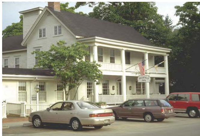
Small scale lodging such as this inn would fit the scale and character of Old Coppell and fill a city-wide need for alternative overnight accommodations.
