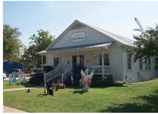
The Old Coppel Gift Shop and the Art Annex are an example of the successful reuse of older buildings.
