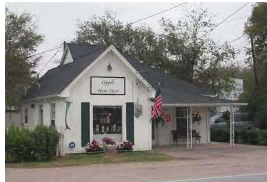
The predominant roof form should be a gable. Gable ends fronting the street are particularly appropriate based on historic precedents in Old Coppel.
