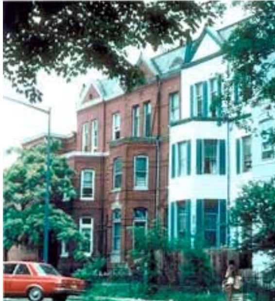
Setting altered by vinyl siding (Taken from the Secretary of the Interior's Standards for Rehabilitation)
