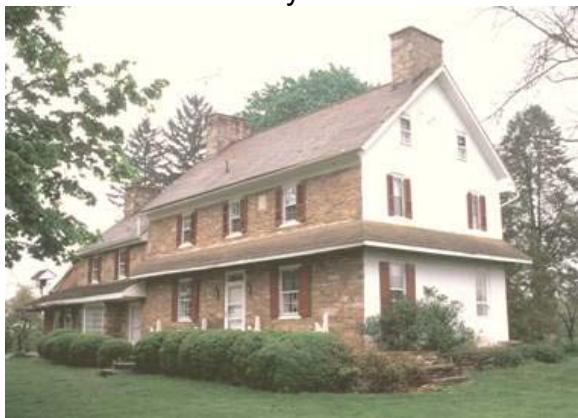
Kitchen addition on left side of building (Good example of an addition being subordinate to main structure)
