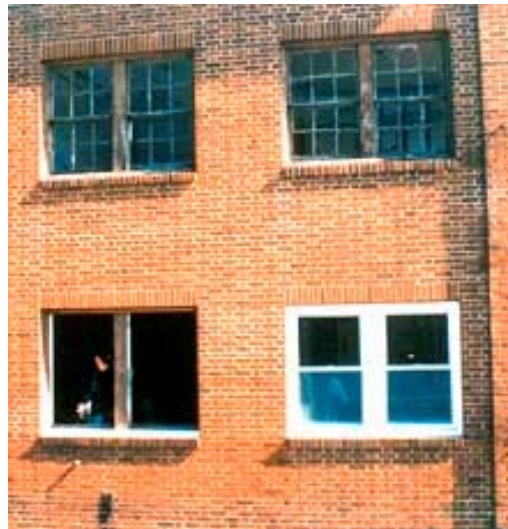
Inappropriate Window change (Taken from the Secretary of the Interior's Standards for Rehabilitation)
