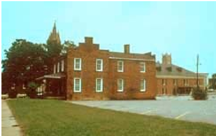
Inappropriate alteration of a site for parking (Taken from the Secretary of the Interior's Standards for Rehabilitation)
