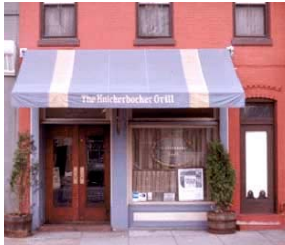
Awning used to reduce heat gain (Taken from the Secretary of the Interior's Standards for Rehabilitation)
